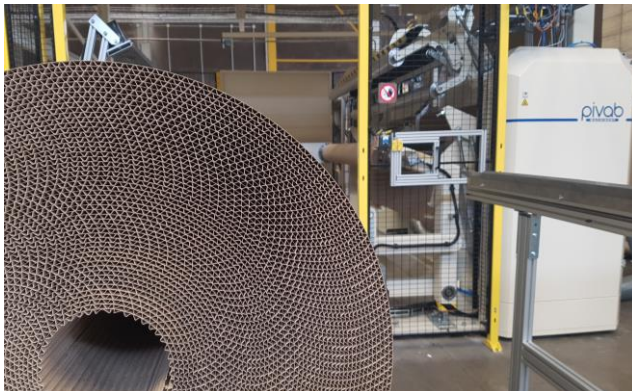
New installation of Pivab rewinder SFC 2583 2.5m at Cartonneries de Gondardennes, France.
